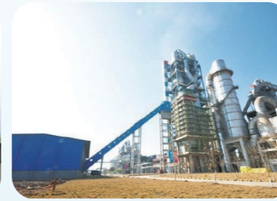
水泥窑协同处置设施 Cement kiln co-processing facility
